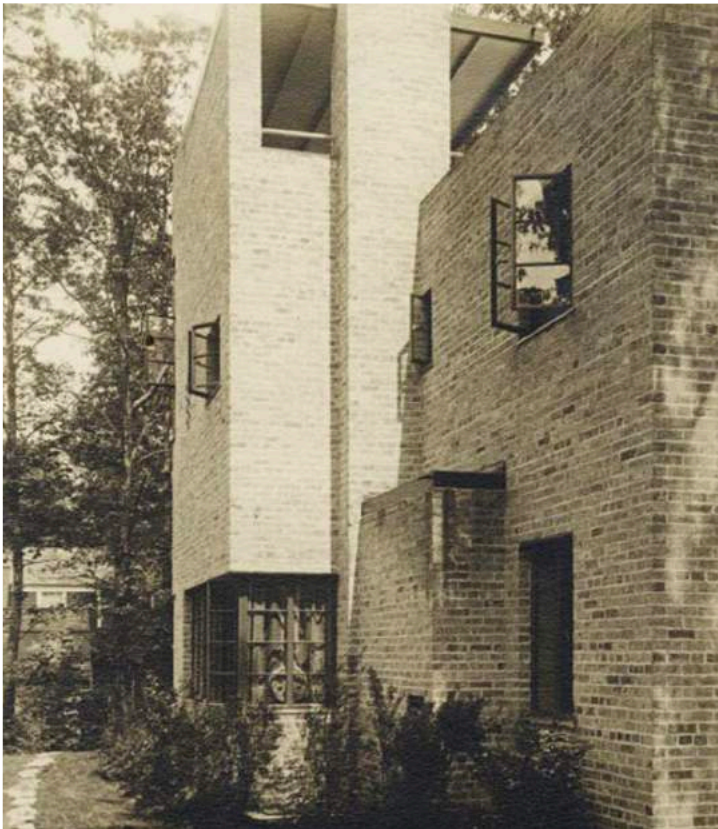
North (rear) facade showing windows to dining alcove and roof terrace canopy.
