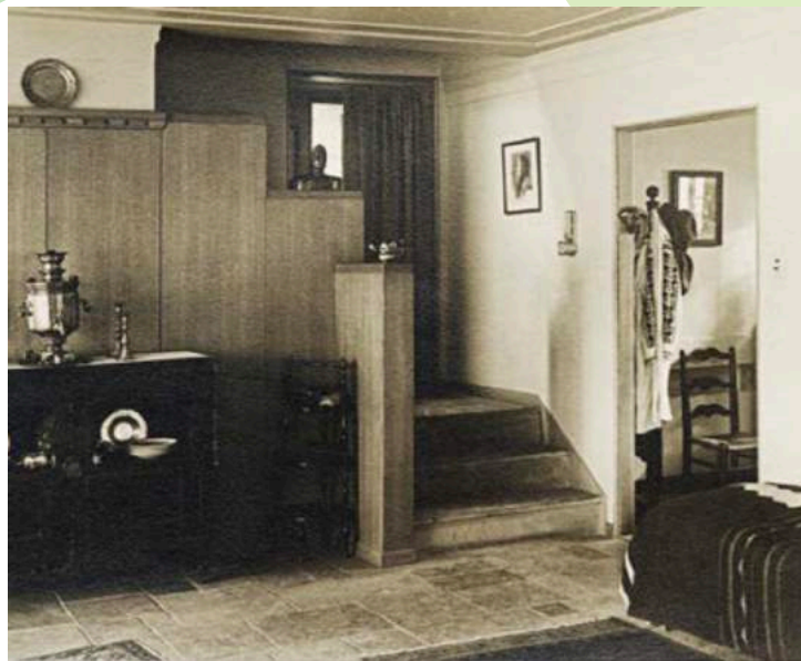
Staircase off of the front entrance.
