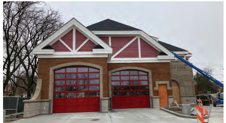
14-foot-wide doors assure quick, safe movement in and out for apparatus. (Photo credit: Jeff Stern)
