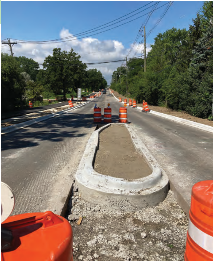
Final blacktopping, scheduled for completion in September, will feature a safety island for pedestrians crossing Clavey between Hillside Dr. and Hastings Ave. (Photo by Jeff Stern)
